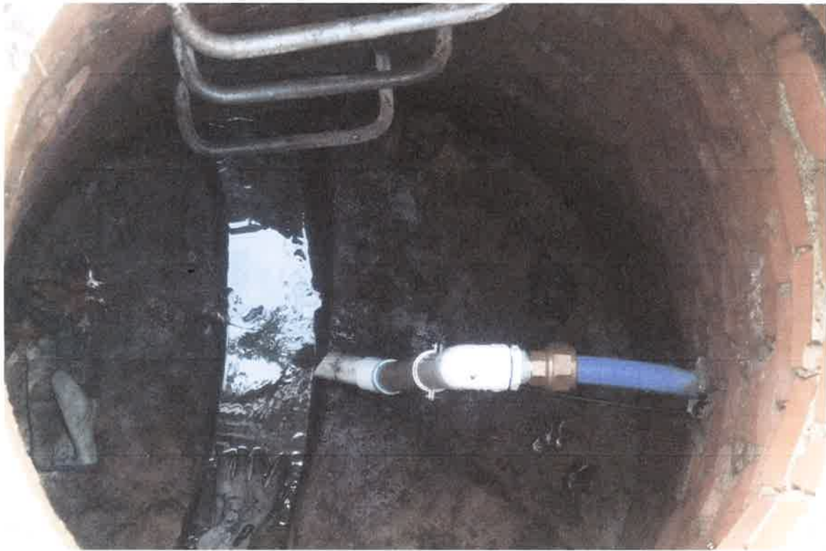
EXAMPLE 11A DROP CONNECTION
