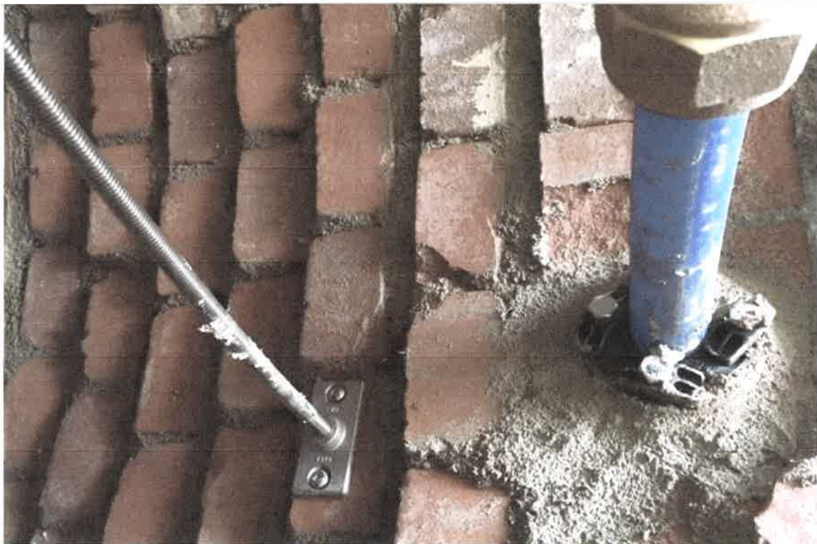
EXAMPLE 11A DROP CONNECTION
